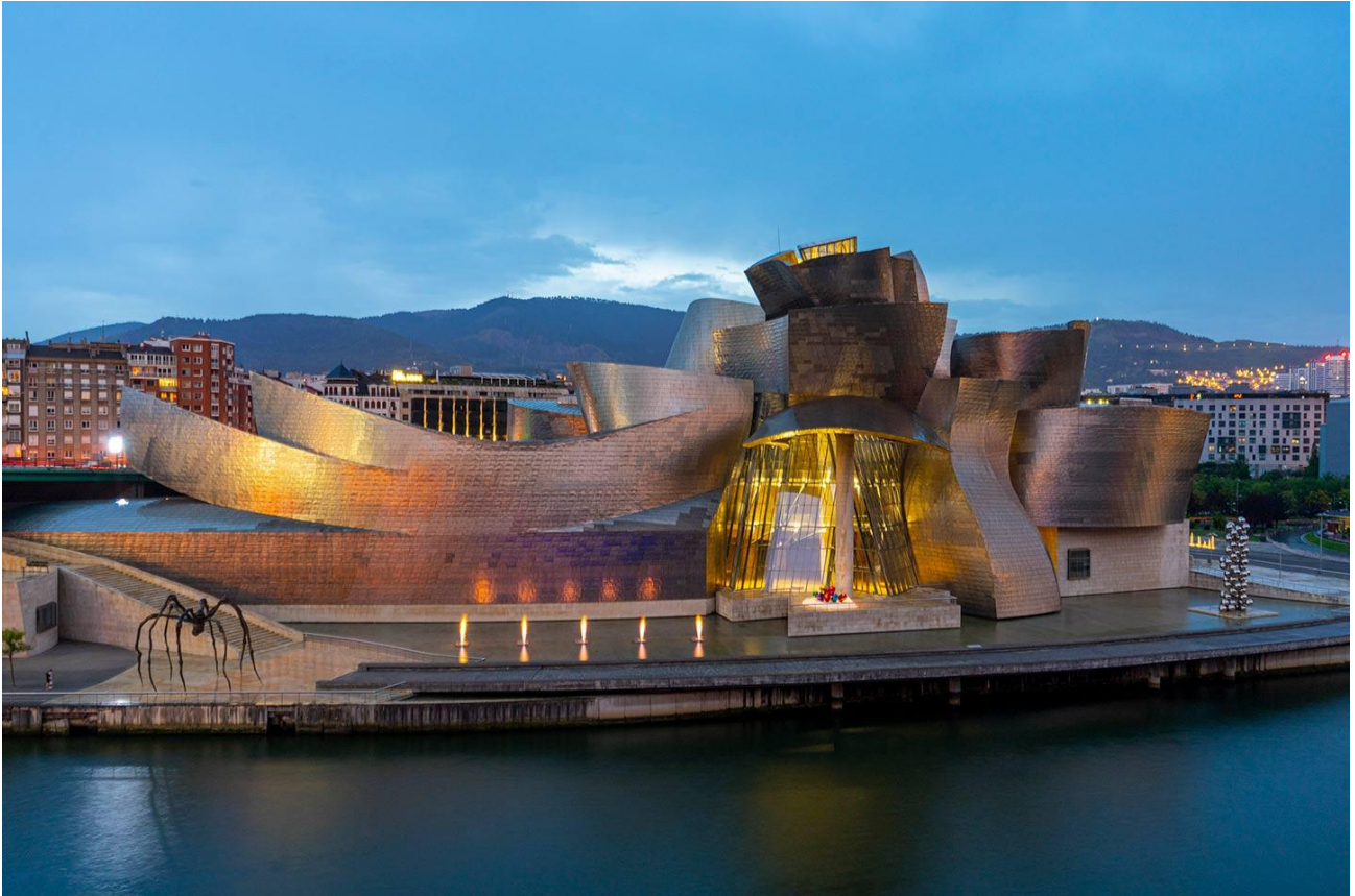
Fig. 6. Guggenheim Museum Bilbao, Spain.
